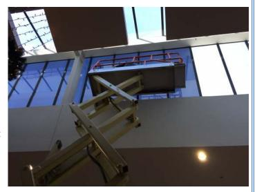
These windows are 2.8 m drop and are 10 metres up from the Shop floor, so nearly 13 metres to top. Because of the close proximity to the Ocean and strong winds blowing salt spray, installing exterior film was not an option, even though we had easier access. The glass was single glaze, toughened safety glass.
